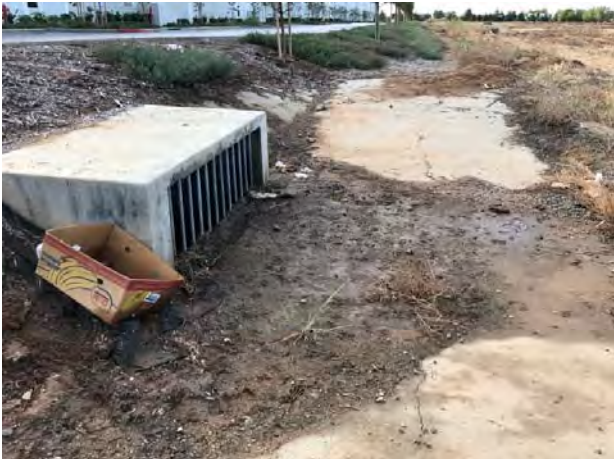
11.View of the stormwater drain on the south boundary.
