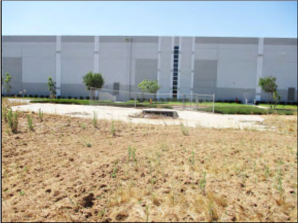
Photo 2: View of Concrete inlet at terminus of Drainage A.
