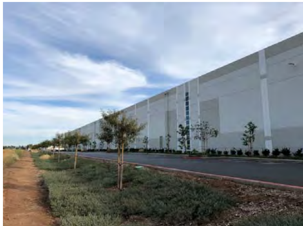
18.View of the landscaped areas on the south and adjacent warehouse building.
