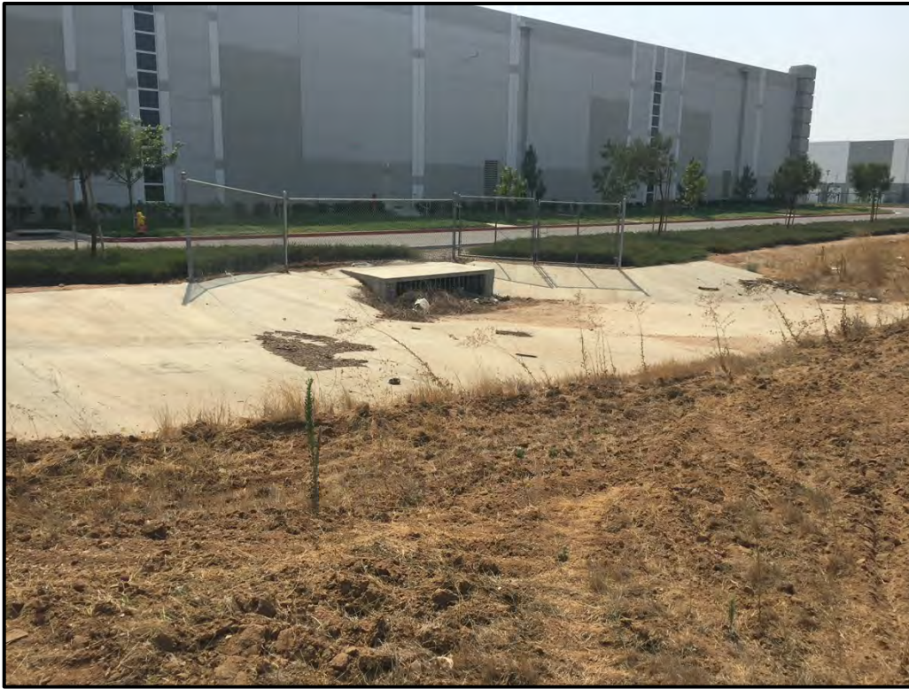
Plate 5.2–4: View of a storm drain found along the southern boundary of the subject property, facing south.
