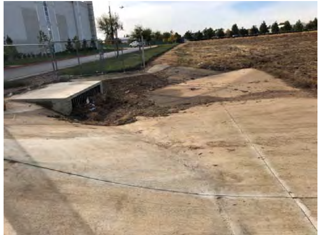
12.View of the southwest stormwater drain on the south boundary.
