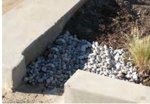
Figure 2: Curb Cut located in a Bioretention Facility
