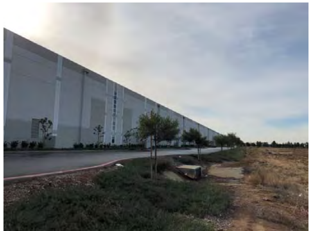
10.View of the stormwater drain on the south boundary.
