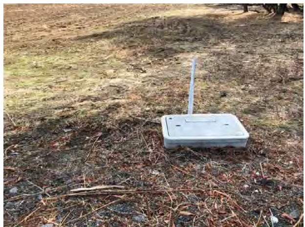
4.View of the communication utility boxes on the north boundary of the subject property.
