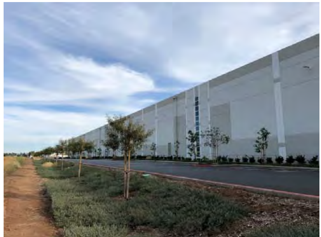
18.View of the landscaped areas on the south and adjacent warehouse building.
