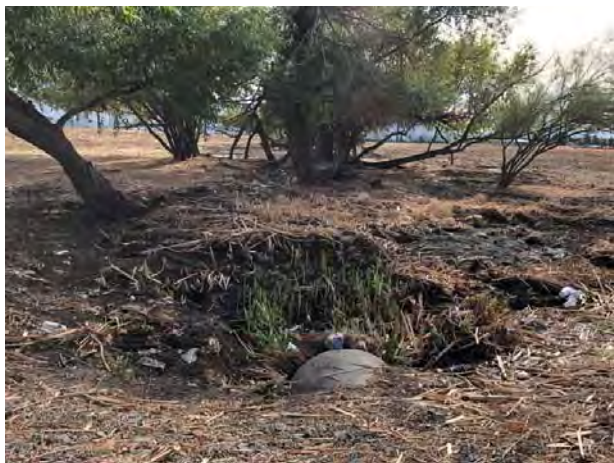
5.View of a storm water drain (easement) draining onto the subject property.
