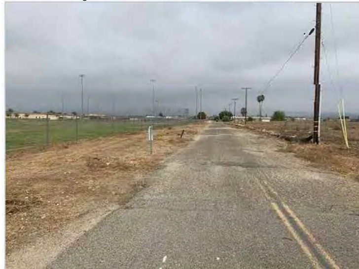
PHOTO 5 North at Emma Lane
