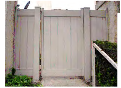
VINYL FENCE AND VINYL GATE
