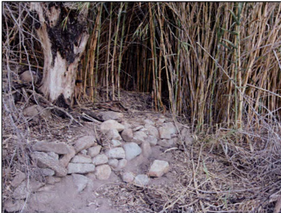
Photograph 2: Dry laid wall
