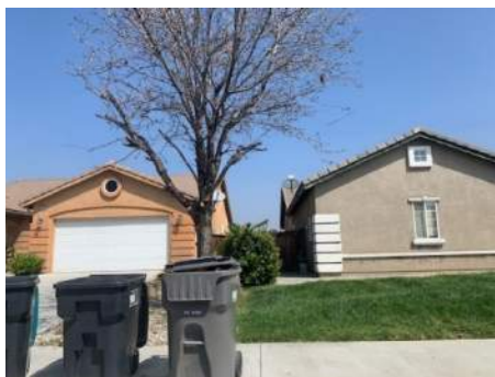
P4- Surrounding Homes South of the Project Site (R5 Zoning) pt.4
