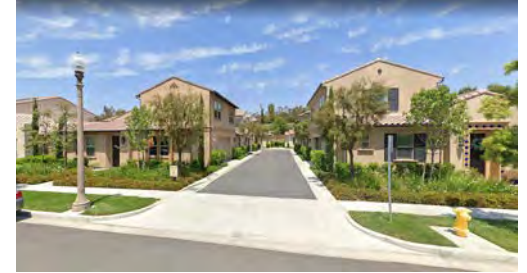
Example of Buildings fronting the Street
