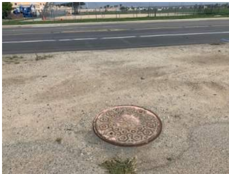
P19- Sewer Connection on the street perimeter of Iris Ave.
