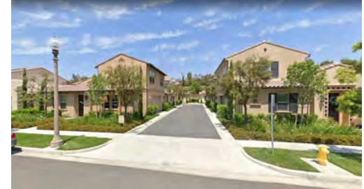
Example of Buildings fronting the Street
