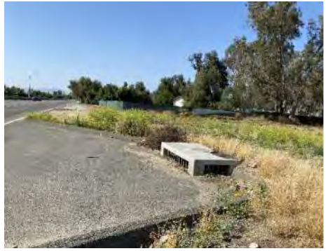
Photo 18: From Indian Street looking north towards an existing drainage inlet along the western boundary of the Project Site.
