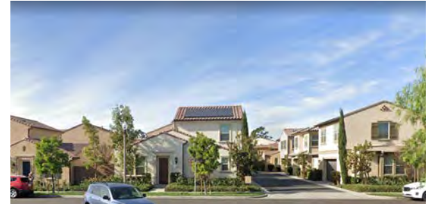
Example of Varied Elevations to Create an Interesting Streetscene
