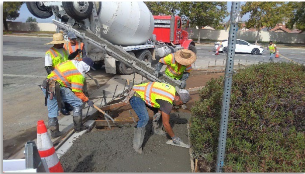
Citywide Pavement Rehabilitation | Moreno Valley, CA
