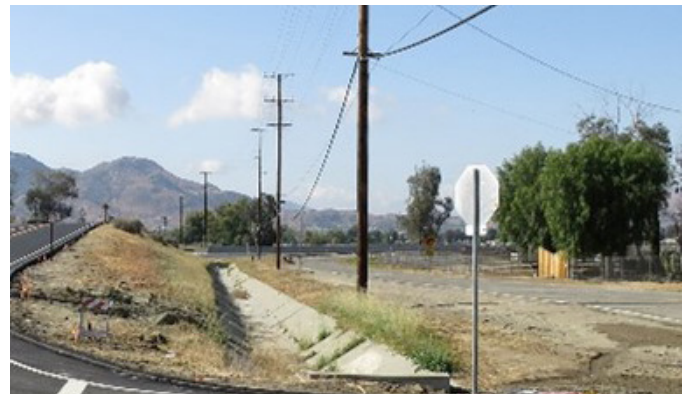
Existing SCE OH Lines & RCFCD Concrete Channel.
