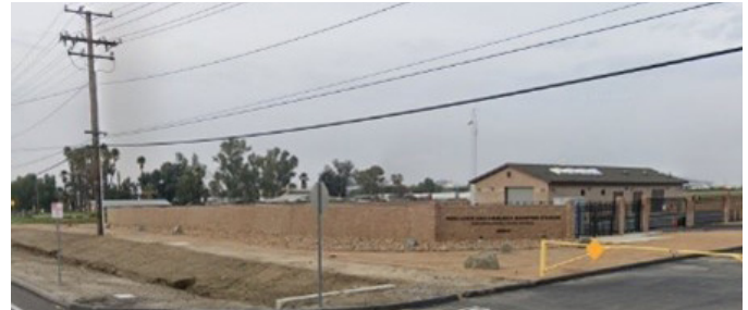
The Existing Redlands / Hemlock EMWD Booster Station. Protect in Place and Coordinate New Utility Lines.
